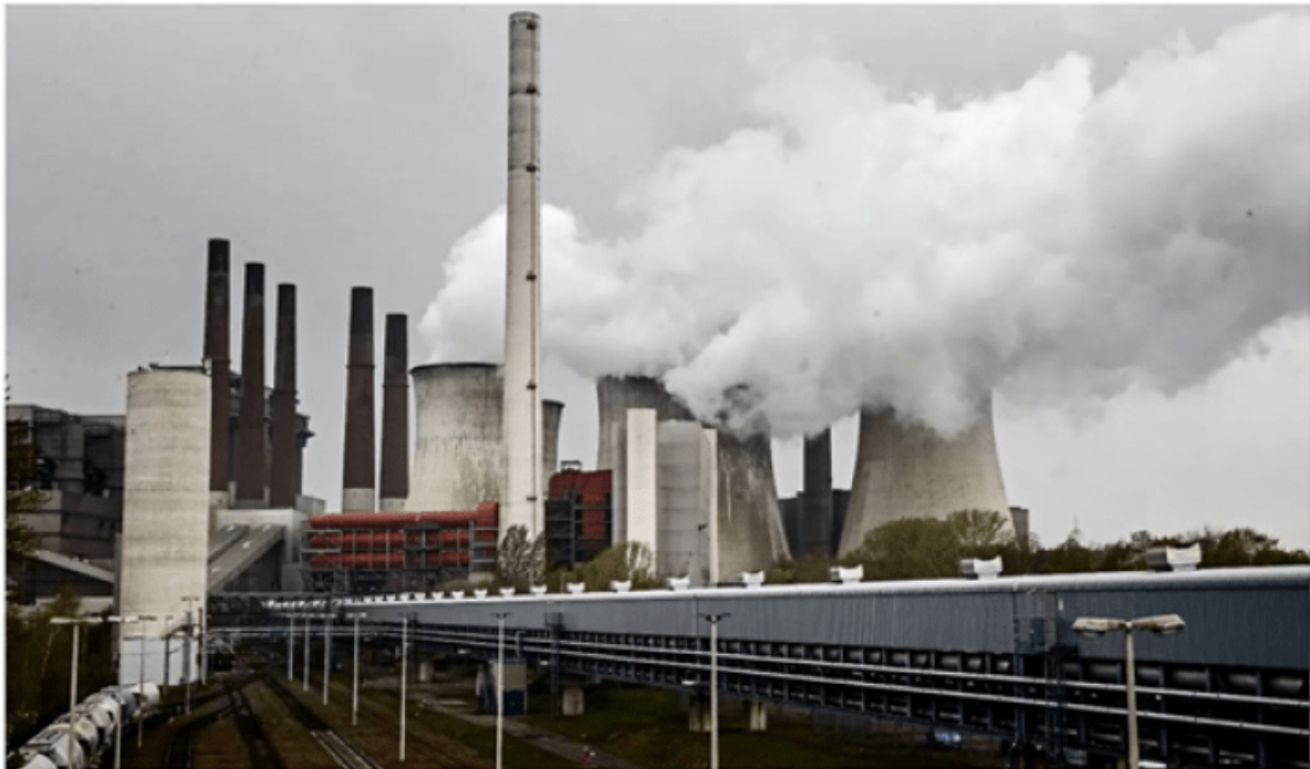
A coal-fired power plant in Germany. A United Nations climate report warns that global warming is on track to exceed 1.5 degrees Celsius by the early 2030s without swift reductions in greenhouse gas pollution. (Martin Meissner / Associated Press )
