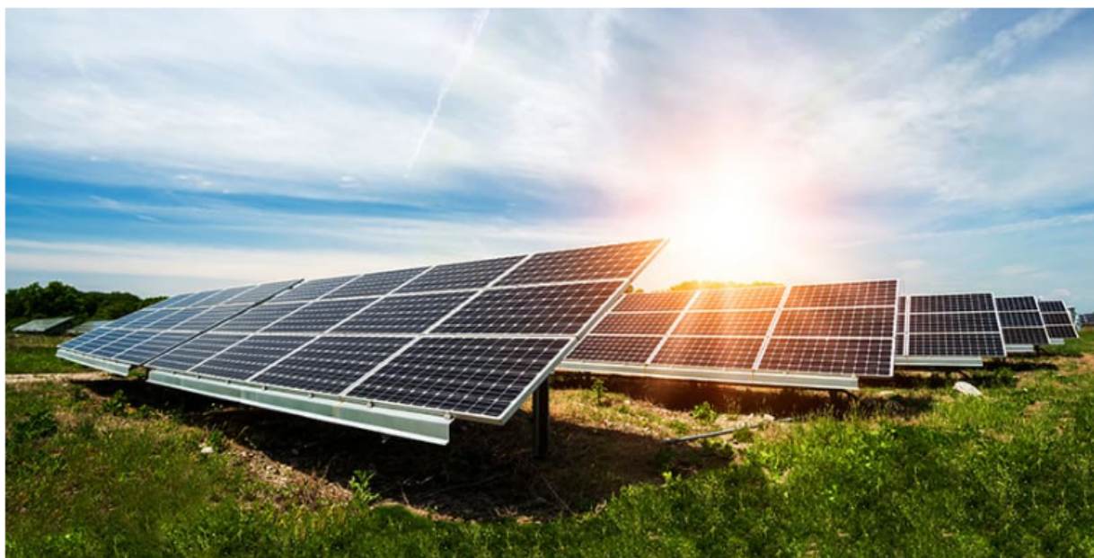
Solar panels in field with the sun reflecting on the panels creating a glare
