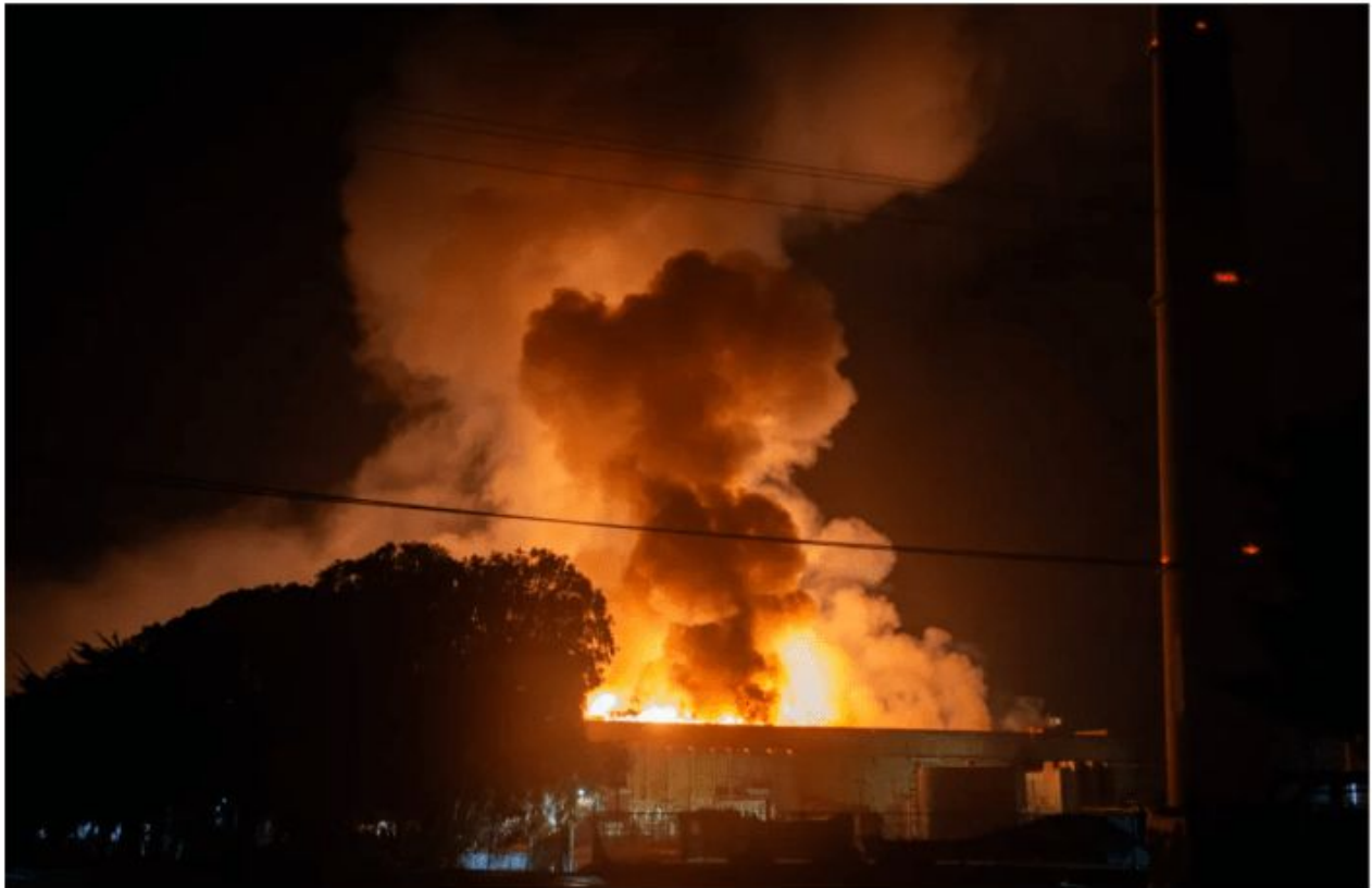
A fire rages out of control at the Vistra battery storage plant, one of the world's largest, in Moss Landing, Calif., on Thursday, Jan. 16, 2025. (Doug Duran/Bay Area News Group)
