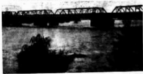
Rising floodwaters inundated the river at 11:00 a.m. on Monday night, which was the highest water level since the 1958 flood. The water was 23 feet 6 inches above the bridge deck. The water was 23 feet 6 inches above the bridge deck.
