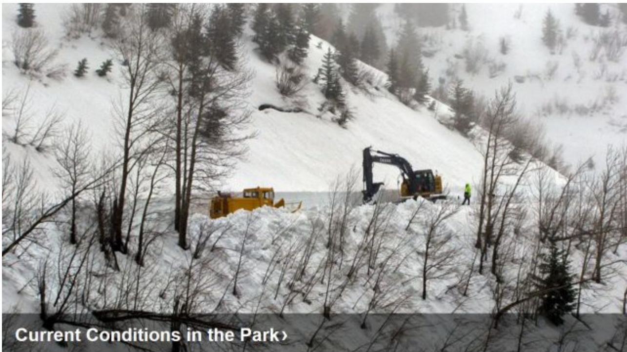
Crews are active working to reopen the Going-to-the-Sun Road
