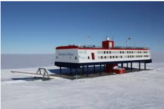
Neumayer III Station
