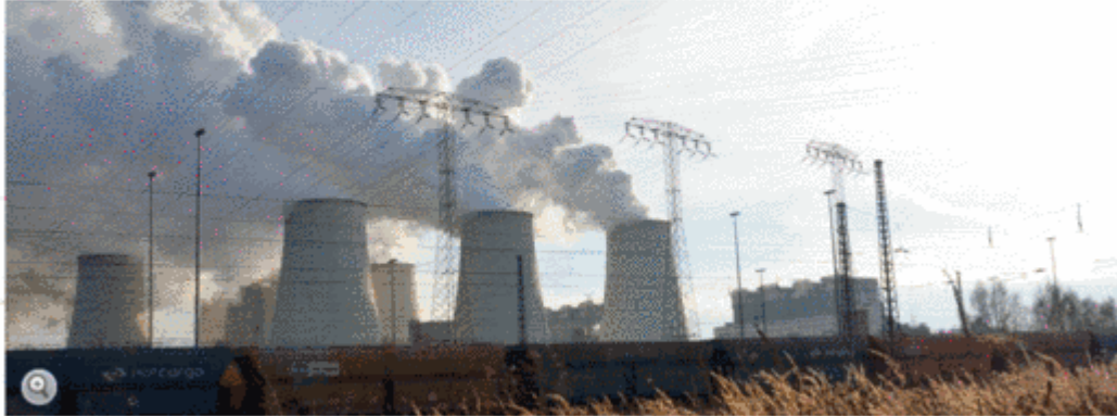
A coal-fired power plant in Brandenburg.
